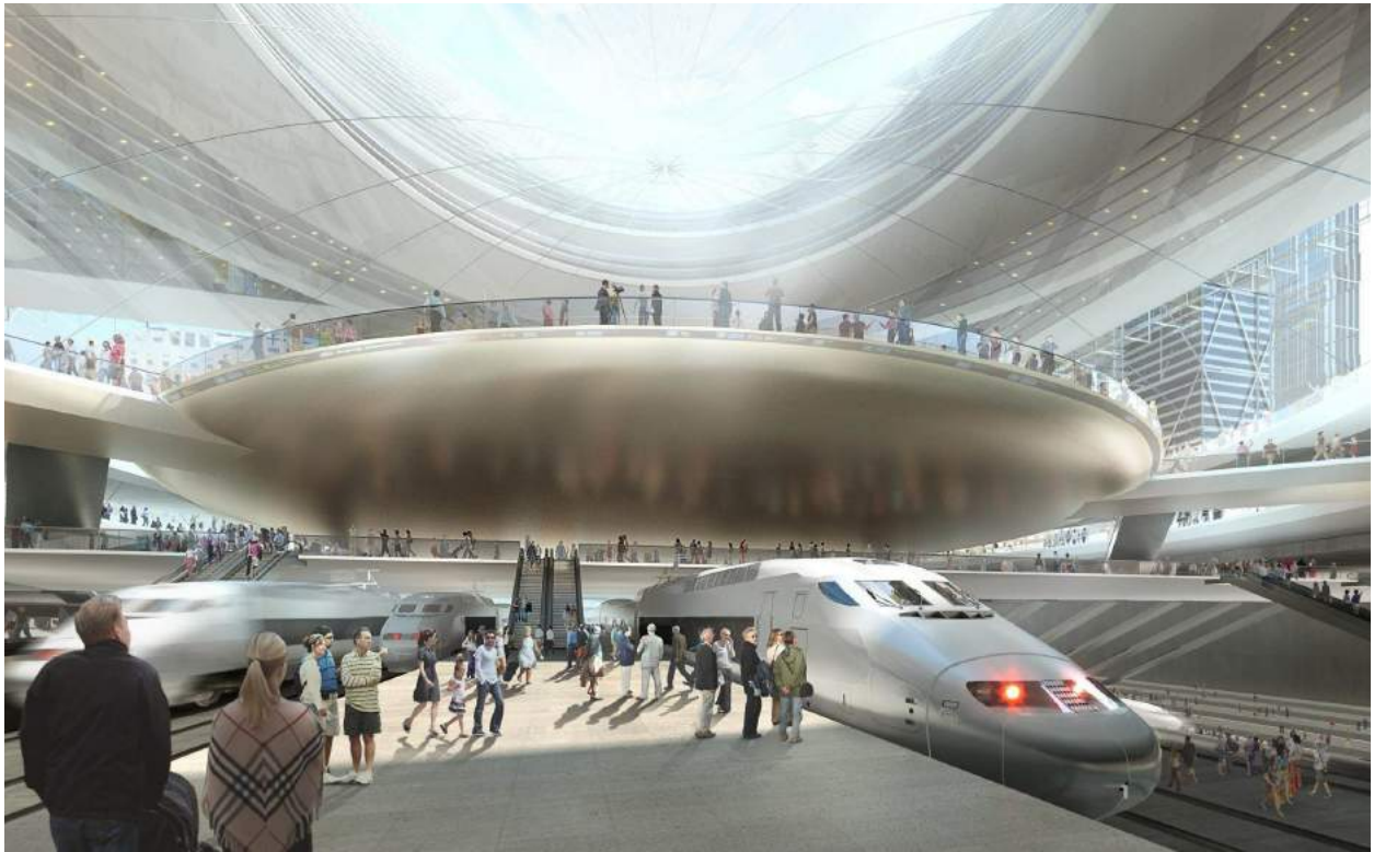
Proposed platforms free from columns. Courtesy of SOM
