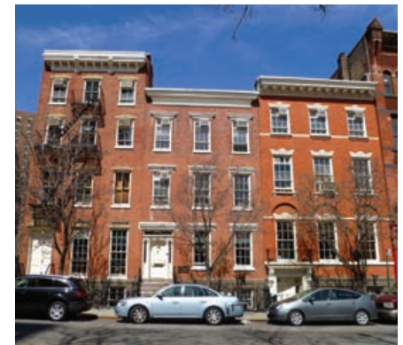
Facades of 263, 265 & 267 Henry Street. The project team's holistic approach to achieving sustainable operations focused on resource use reductions in the building design, as well as building operations and user behavior.
