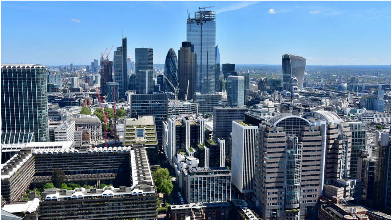
City of London under construction (Source: Flickr, The Commons, Michael Gwyther-Jones)
